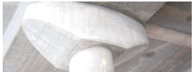
Self Compacting Concrete (SCC)
