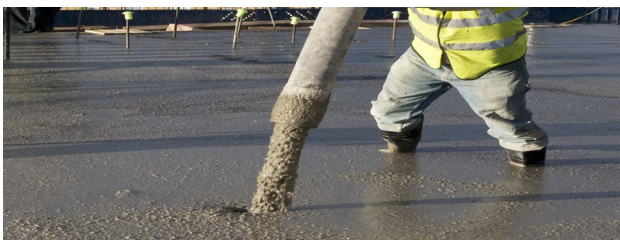
Pumped Concrete
