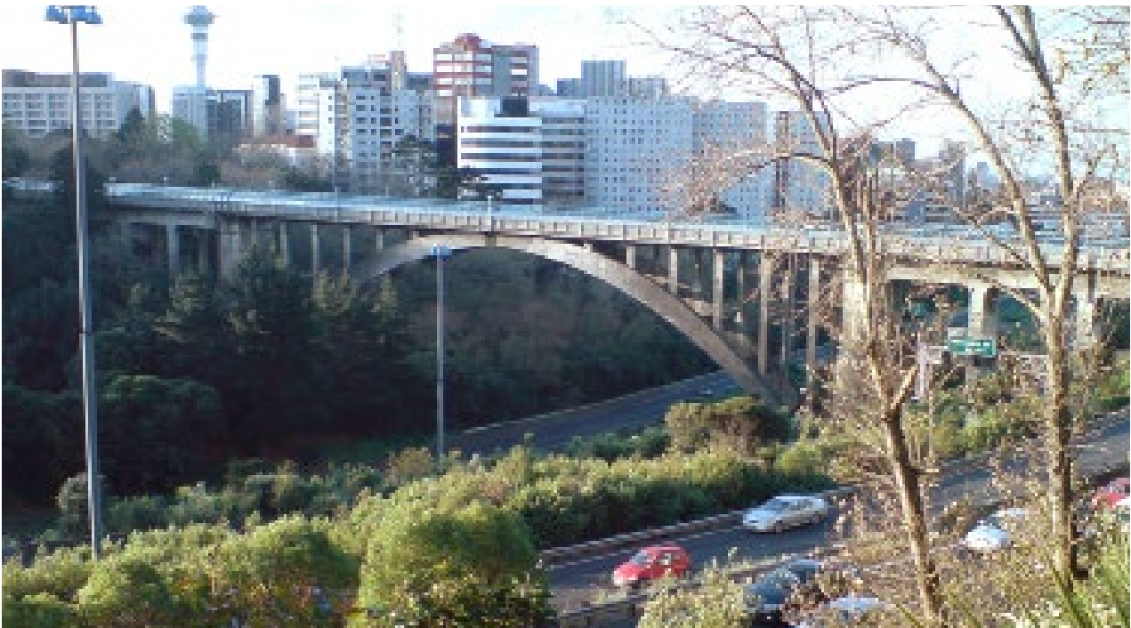
Grafton Bridge, Auckland, New Zealand
