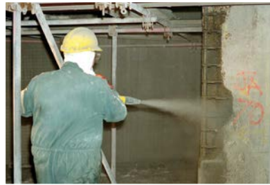
Machine applied concrete repairs
