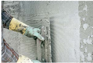
Hand applied mortar
