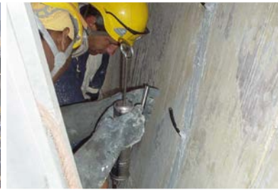
Watertight crack sealing by injection
