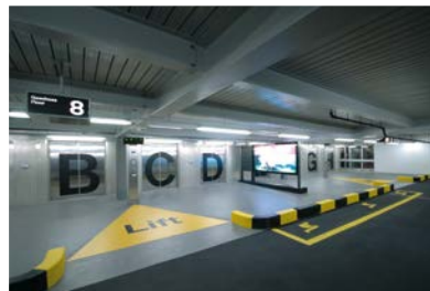
Flooring in car park decks
