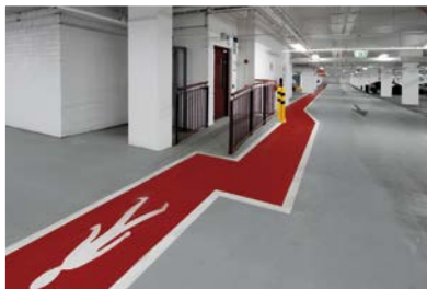
Flooring in car parking areas
