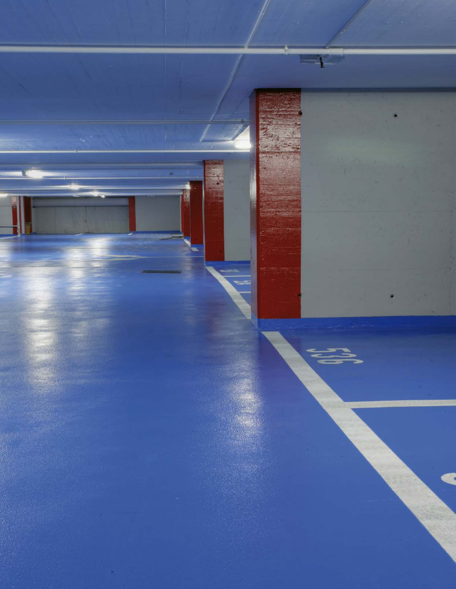
Hotel Novotel, Switzerland 3300m 2 of Sikafloor ® solution were installed in the car park of the Novotel Hotel in Geneva.
