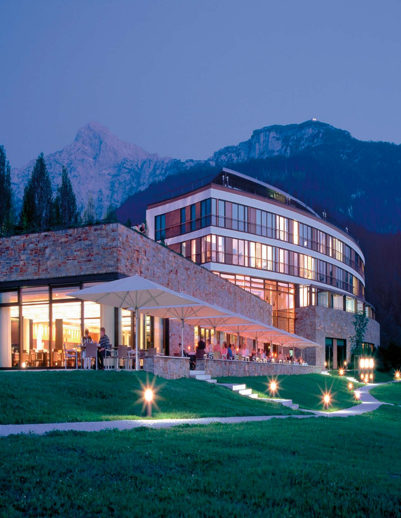
Resort Hotel Intercontinental, Germany In order to avoid contamination from the kitchen into the rooms below - 1000 m 2 Sikaplan ® membranes were installed beneath the tiles in the kitchen.
