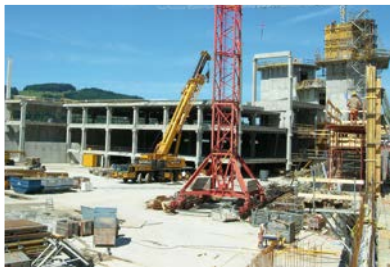
Site batched concrete production
