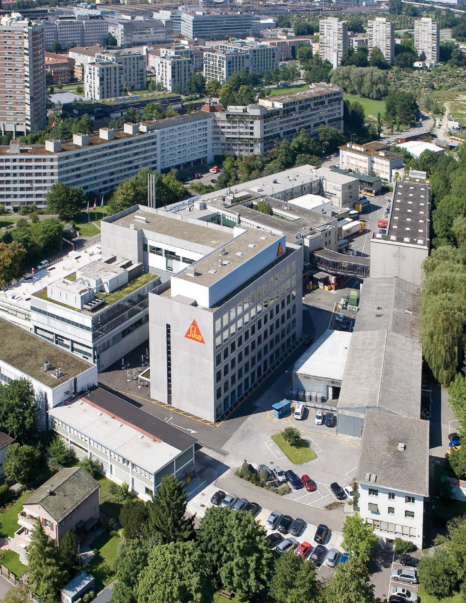
The headquarter of Sika Switzerland Zurich, Switzerland
