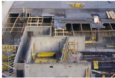
Watertight concrete for basement waterproofing
