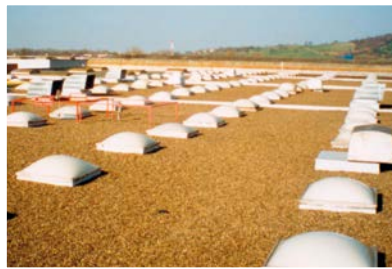
Roofing for gravel ballasted roofs
