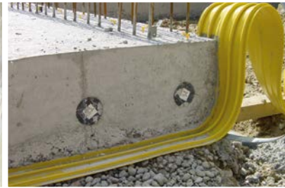
Waterstops for integral joint waterproofing
