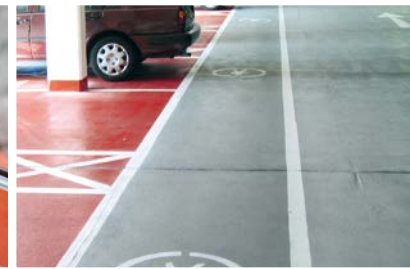
Sealing of floor joints in carpark and elsewhere
