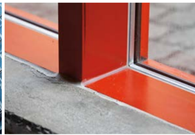
Sealing of connection joints around windows and doors
