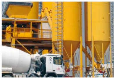
Ready-mix concrete production
