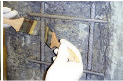
Protection of steel reinforcement
