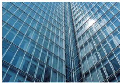
Sealing of glas façades
