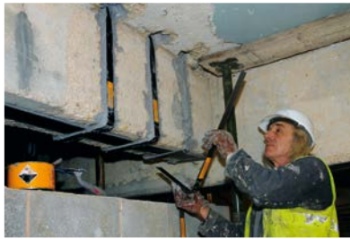
Shear strengthening of beams
