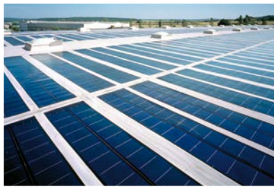
Roofing for solar roofs
