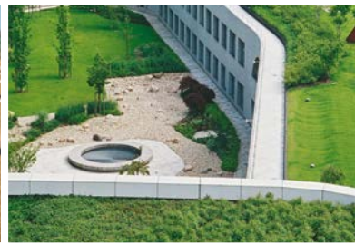
Roofing for green roofs
