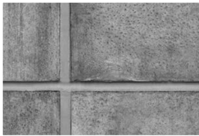
Sealing of stone, brick and concrete joints
